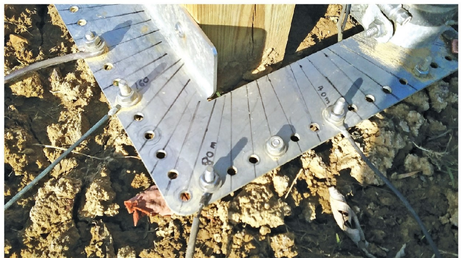
Figure 3 — I laid new radials out in the direction indicated by the marker line, and marked the length of the radial along the marker line. "80 m" indicates that the radial is \frac{1}{4} wavelength long for the 80-meter band. [Mike Conlon, N2EM, photo]
