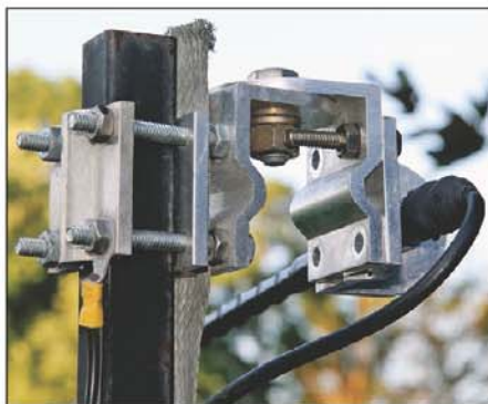
Figure 2 — This arrangement of three CB-style mounting brackets makes for a simple drop-down mount for your vertical antenna. [Mayor Nelson, KD5LBE, photo]
