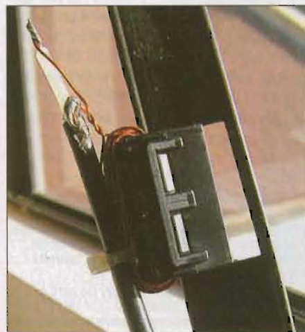
Figure 2 — Here, the snap-on ferrite choke is snapped in place over one of the wires in a piece of window line parallel feed line.
